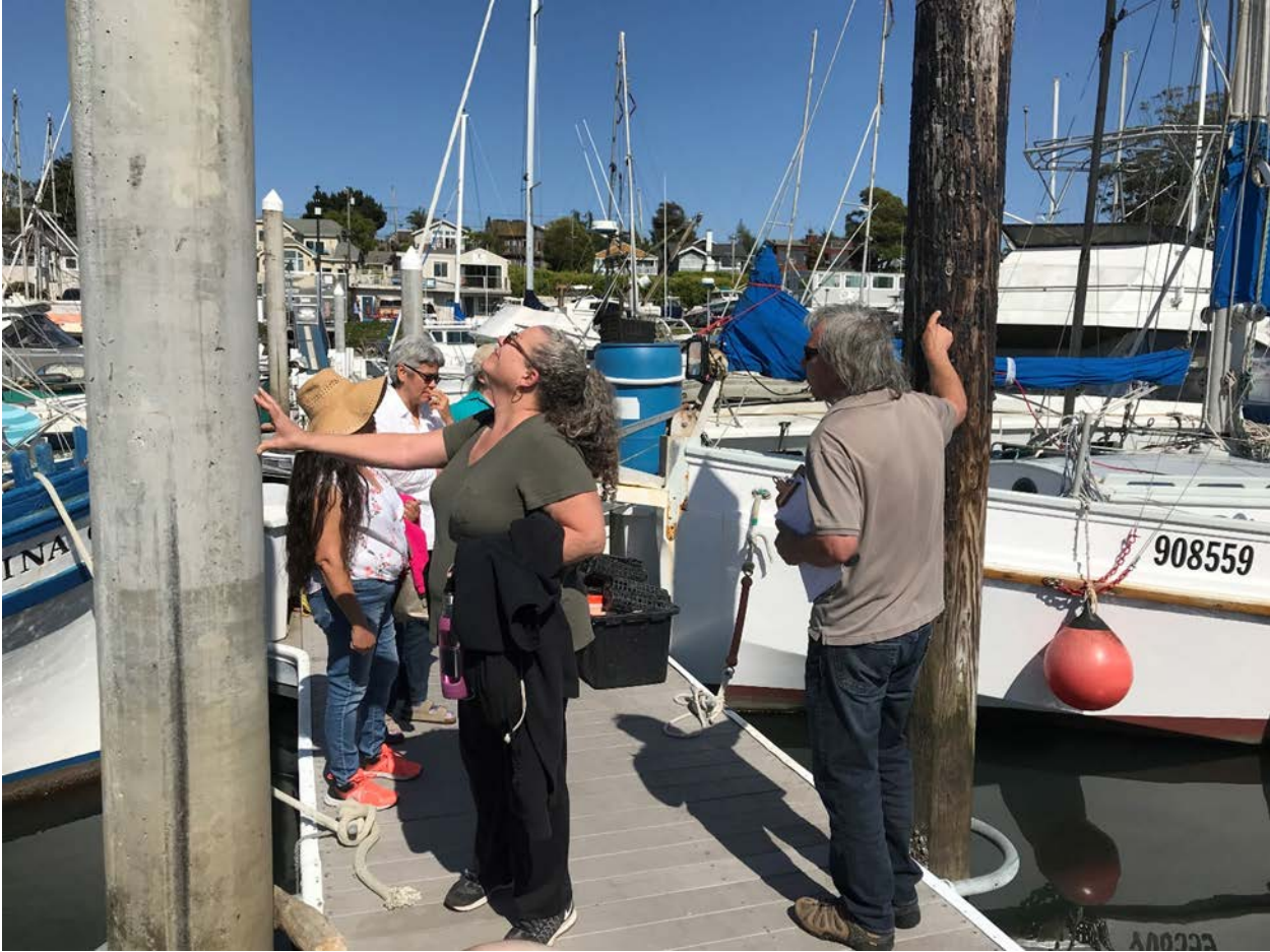
Photo 3: Several generations of piles are apparent in the harbor. The piles associated with the floating docks and other over-water structures were initially creosote-treated Douglas fir, seen on the right.
